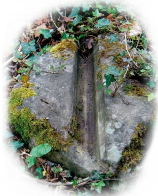
Grooves worn into stone where rope, and later iron cable, rubbed as trucks went up and down.
