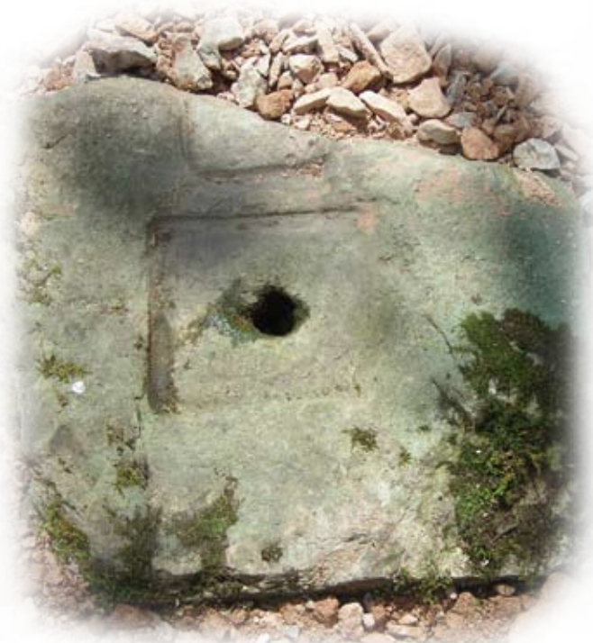
Stone sleepers – the holes were for pegs to fix an iron 'shoe' which held the rails in place.
