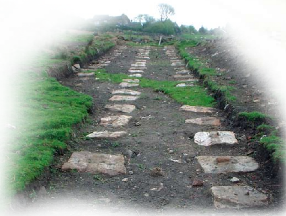
A similar tramway in Derbyshire showing the longitudinal lay out of the stone sleepers.
