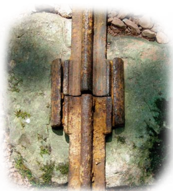
The original rails were cast iron with a cross section of an upside-down T – they had a tendency to break near the join. The truck wheels had a flange on each side.
